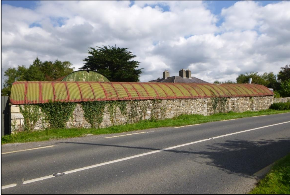
Plate 6 View NE to linear outbuilding range at Confey House from entrance into proposed LRD on R149.
