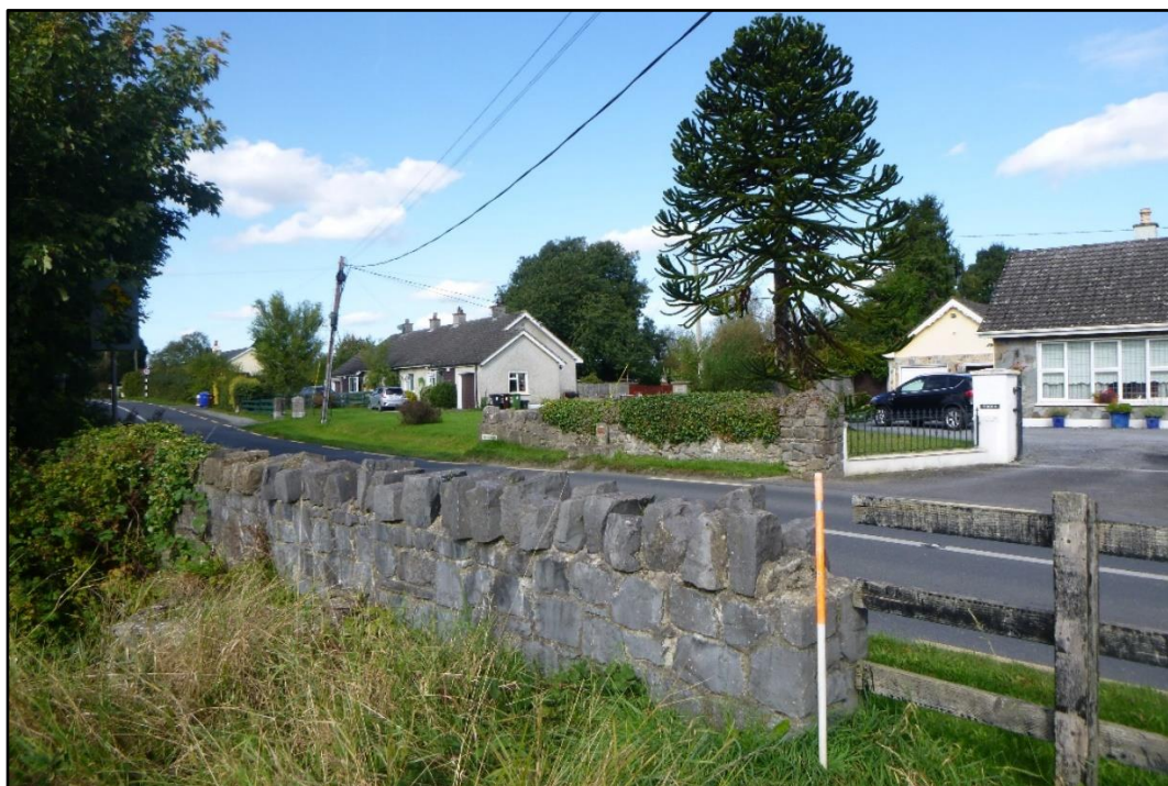
Plate 9 View NW from inside NW corner of proposed LRD to rebuilt bridge side wall on the south side of the R149.
